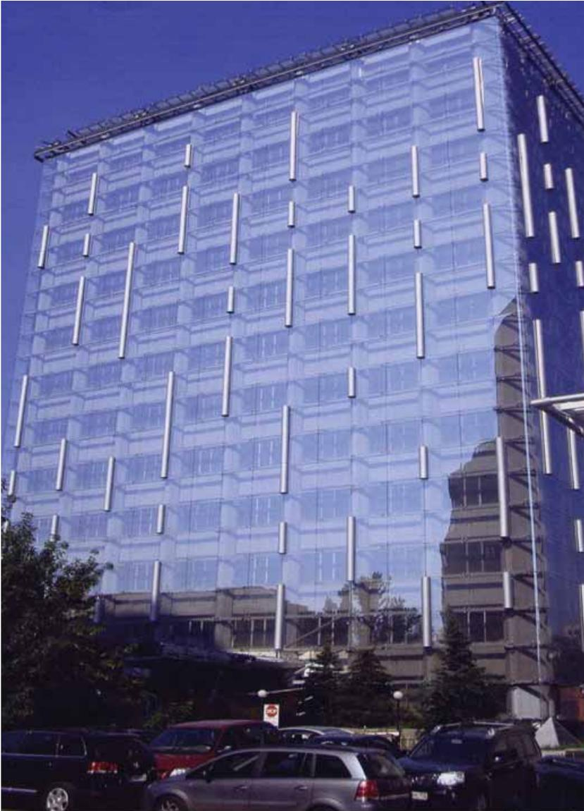
*Figure 7. New image of the old-style building (building with double – skin façade)*
